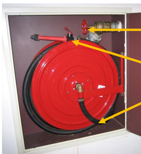
pic.4.4.2: opened wall hydrant cabinet
