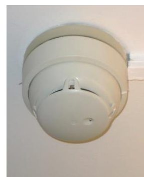
pic. 4.2: smoke detector
