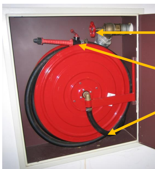
pic.4.4.2: opened wall hydrant cabinet
