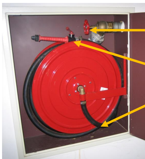
pic.4.4.2: opened wall hydrant cabinet
