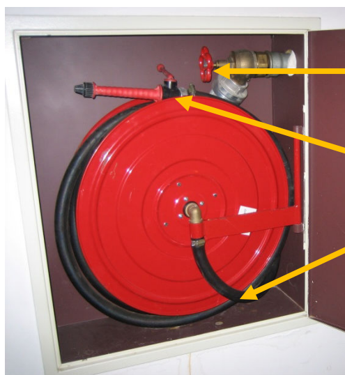
pic.4.4.2: opened wall hydrant cabinet
